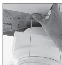
5. Put assembly in place and plumb. Make sure load is centered over column shaft and evenly distributed around the bearing surface. (Column installation kit available #17040)
