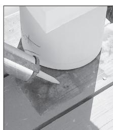
4. Apply construction adhesive\* to top and bottom surfaces of column.
