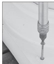
8. Apply construction adhesive\* to bottom of base and nail or screw to floor.
