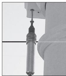
7. Apply construction adhesive\* to top of cap, press against structure, and screw or nail into place.
