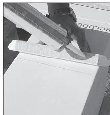
9. Mark location for supplied neck moulding. Measure and cut neck moulding to a 45° angle. Apply construction adhesive\* and put neck mould in place.
