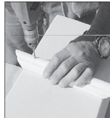
10. Pre-drill holes through neck mould into column. Screw neck mould in place or pre-drill and use finish nails.
