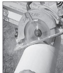
2. Use an abrasive saw (masonry or carbide tip blade). Fine trim top and bottom with rasp to ensure flat surface contact.
