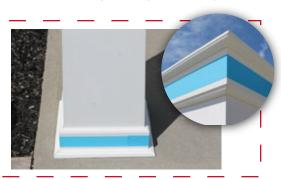
Bottom skirt is now complete! Repeat these steps for the top skirt, and remove support tape once the PVC glue is set.
