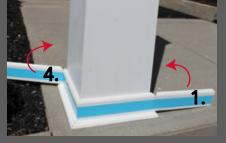
Unfold panels 1 and 4 into final positions. Note that the extra blue support tape can be used to hold the last corner together.
