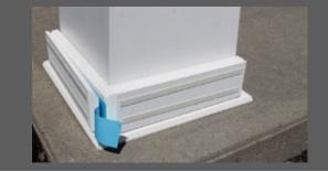
Slide on panel 3 backing position skirt until panel 2 makes contact, then remove backing from panel 3 adhesive strips and press into position.
