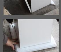
**10.** Fasten the remaining squaring corners into place at the top and bottom, ensuring to use PVC adhesive on one half of each miter.
