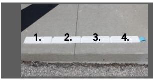
Take backing off the adhesive strips on panels 1, 2, and 4 (keep them on panel 3 to allow for positioning)
