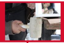
\*A rubber mallet can be used to tap joints into position. Light tapping is all that's needed - do not hit too hard, as corners can fracture.
